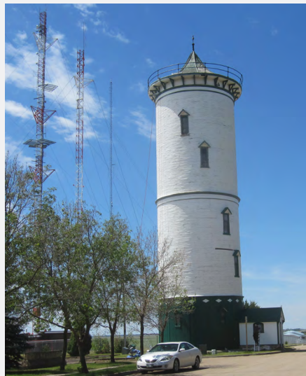
> Weyburn Water Tower, located on 10th Ave. S, besides the TC Douglas Centre.
